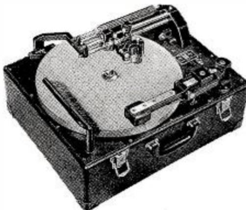
Fairchild Unit 523 is used in fixed studio installations for dubbing sound tracks for motion picture production. Absolute lip synchronism is guaranteed for use with your cameras and projectors. You get this same performance with the portable Fairchild Unit 539-G Disk Recorder shown at left. Many motion picture sound tracks are first recorded on FAIRCHILD SYNCHRONOUS DISK RECORDERS.
