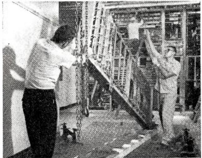
**STEADY AS SHE GOES.** After uncrating, the intricate frames of switching equipment are hoisted upright and placed in position. One hundred ninety such frames are being installed in Vincennes, bringing dial service to over 7,000 telephone customers.
