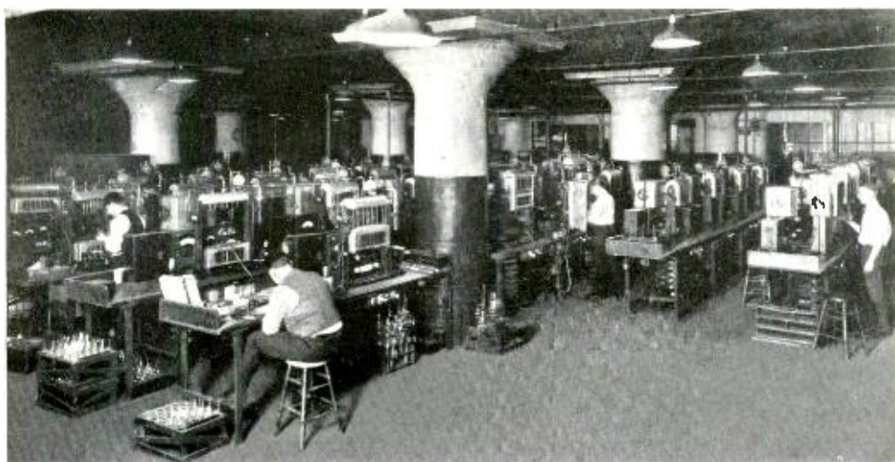
A section of the Vacuum Pump Department
