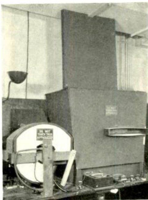
Apparatus for observing reaction between a beam of electrons and a single crystal of nickel
