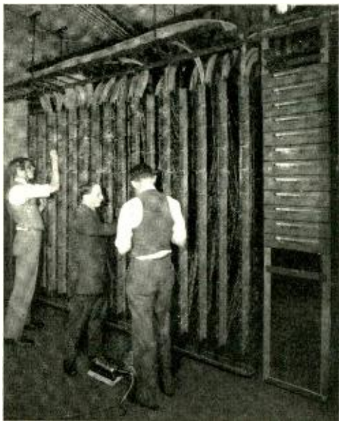
J. E. Devany supervising the work on an intermediate distributing frame
