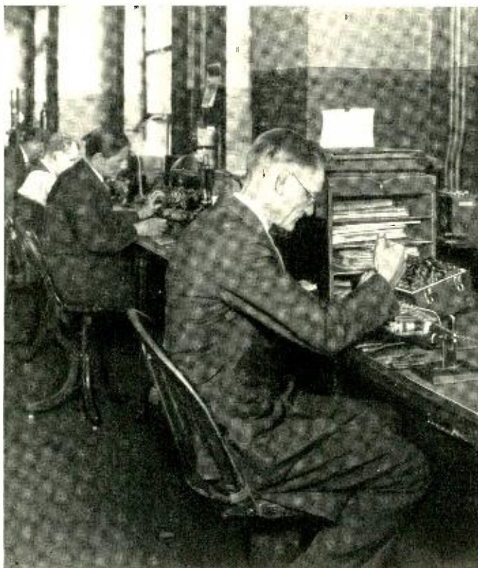
A. Bregartner adjusting a series of "E" type relays
