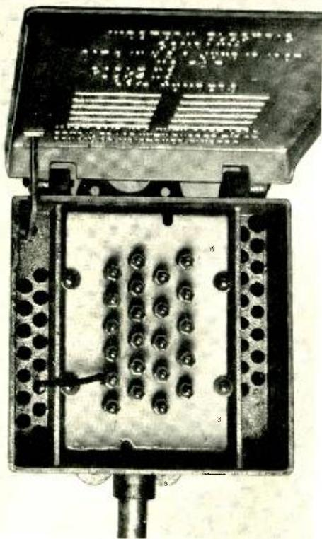
*Fig. 4—No. 14 type cable terminal with porcelain block in place*
