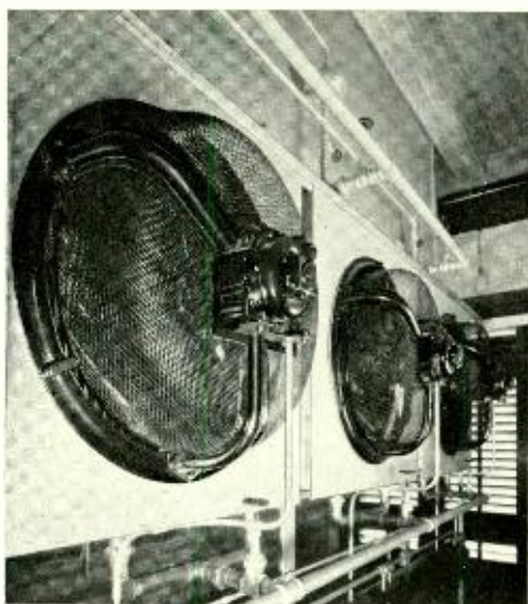
Fig. 6—The three water-cooling units associated with water-cooled vacuum tubes in transmitters and rectifiers
