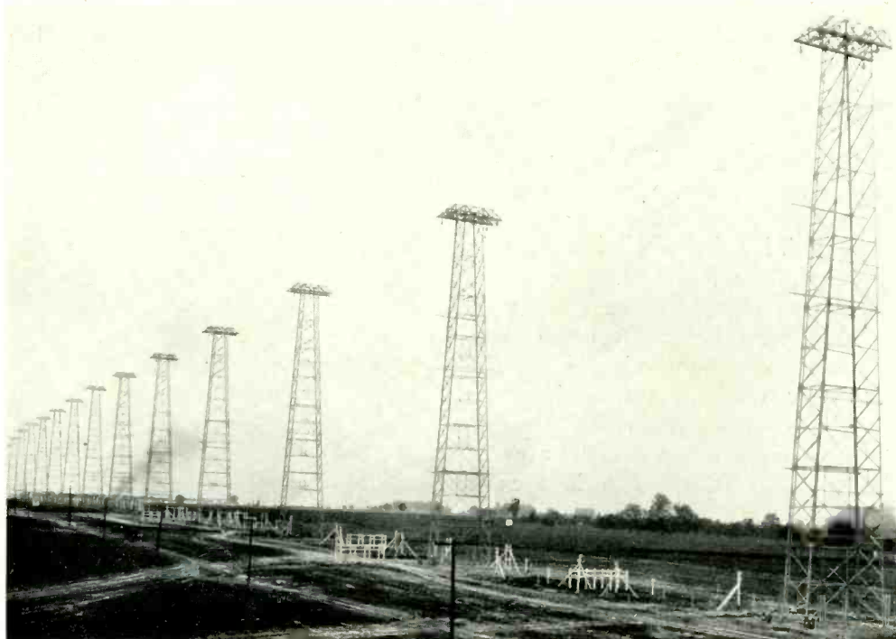
A part of the line of towers supporting the antennas
