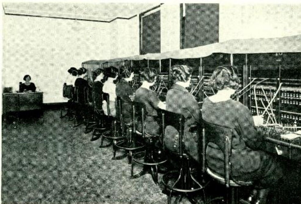
Fig. 3—A medium sized P. B. X. of the manual type is the 600-C
