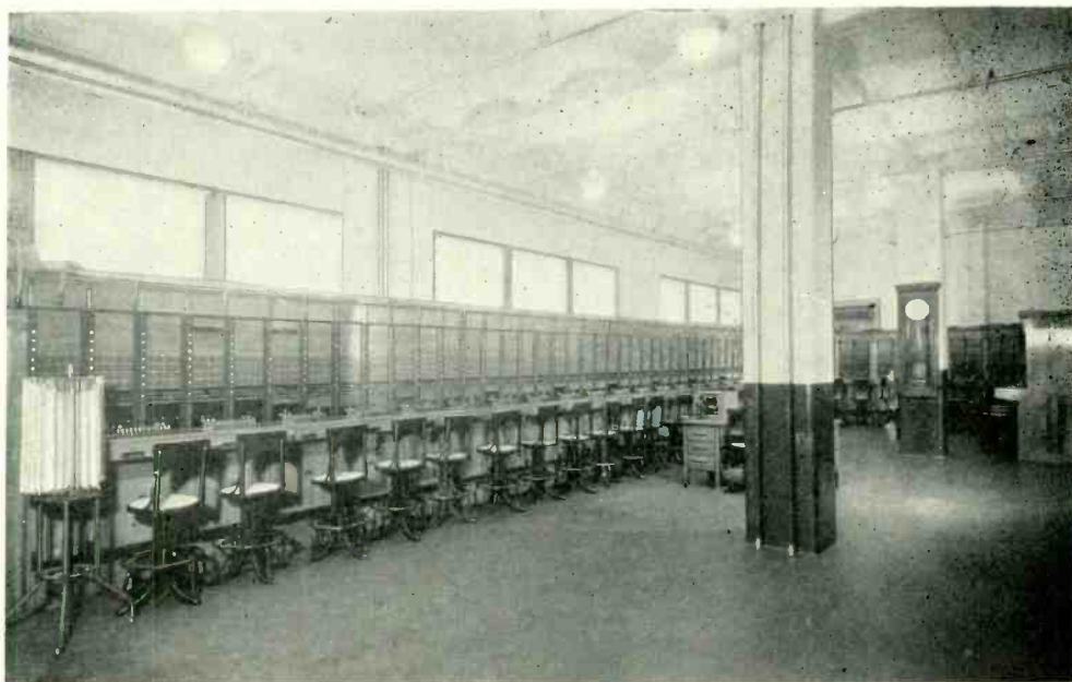
Fig. 2—A large 604-type P. B. X. installed in Bell Telephone Laboratories
