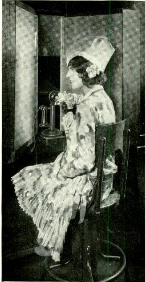
During transmission one sits in front of the apparatus and sees the large sheets of diffusing glass behind which are the color-sensitive photoelectric cells
