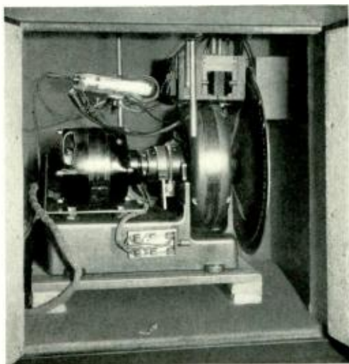
The disc and motor drive for the color television apparatus are the same as for monochromatic television. The mirror and colored filters are in the small box behind the disc. One of the water-cooled argon lamps appears above the motor
