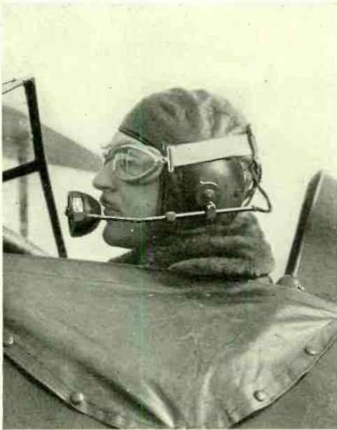
Fig. 4—For single seat mail planes a lighter type of microphone is used, fastened to the aviator's helmet
