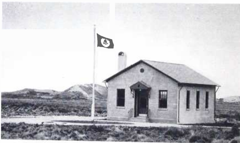
The initial building unit at the transpacific receiving center, Point Reyes, California
