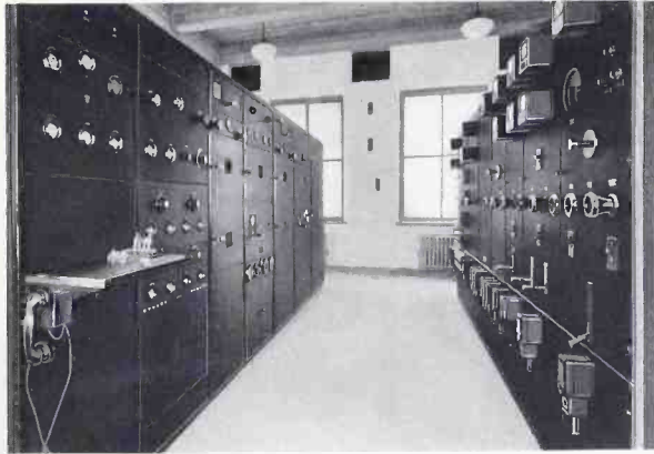
Fig. 3—The transmitter (left) and power control equipment (right) for transmitting to Honolulu are similar to those at Lawrenceville.
