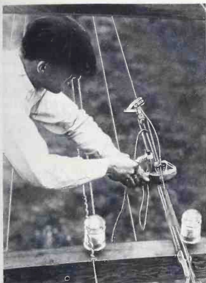
Fig. 5—Making a rolled joint aloft
