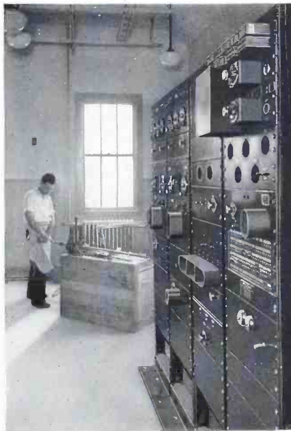
Fig. 6—Installing the receiver at Point Reyes for reception from Honolulu
