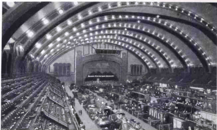
In a gondola above and in front of the stage of the auditorium are located the projectors for stage performances
