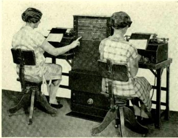
Fig. 2—A broadcasting PBX for printer service with two operators and keys for 24 radial lines
