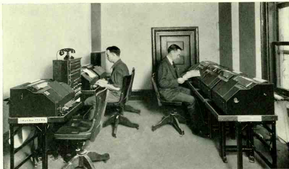
Fig. 3—PBX for printing telegraph system in headquarters' office of the Borough of Manhattan
