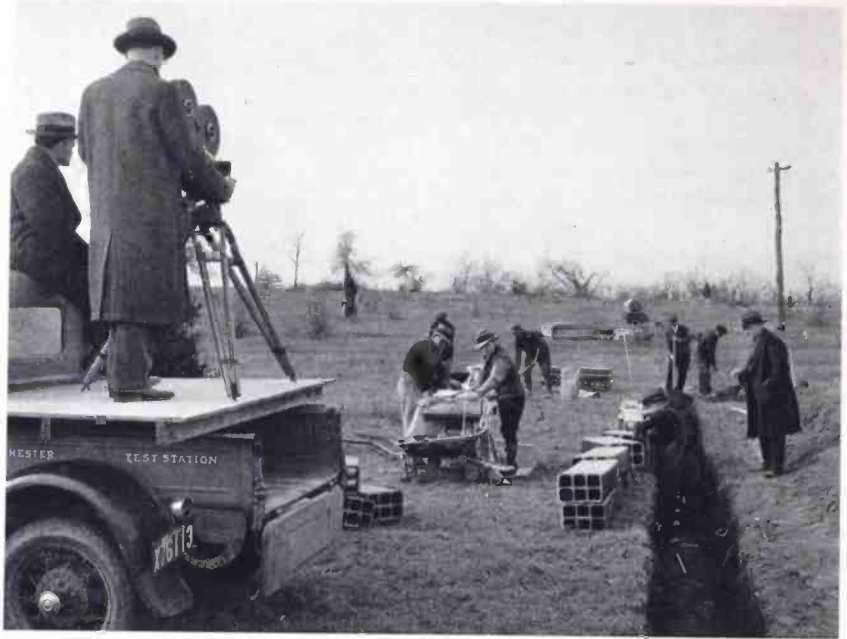
Fig. 4—Taking a motion picture illustrating the making and applying of mortar bandage joints to serve as instructions to the field
