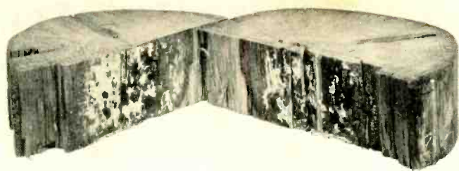
Fig. 7—This section of a decayed test specimen shows the matted structure of a fungus growing within the wood
