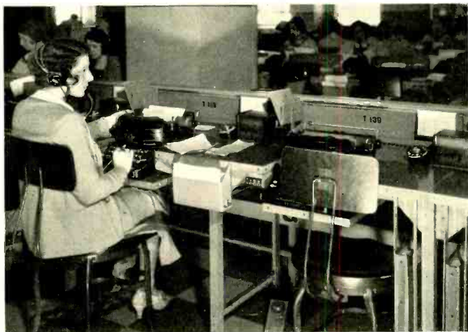
Fig. 3—From a position equipped with four keys outside calls may be made. This enables the attendants at these positions to deliver messages as well as to receive them
