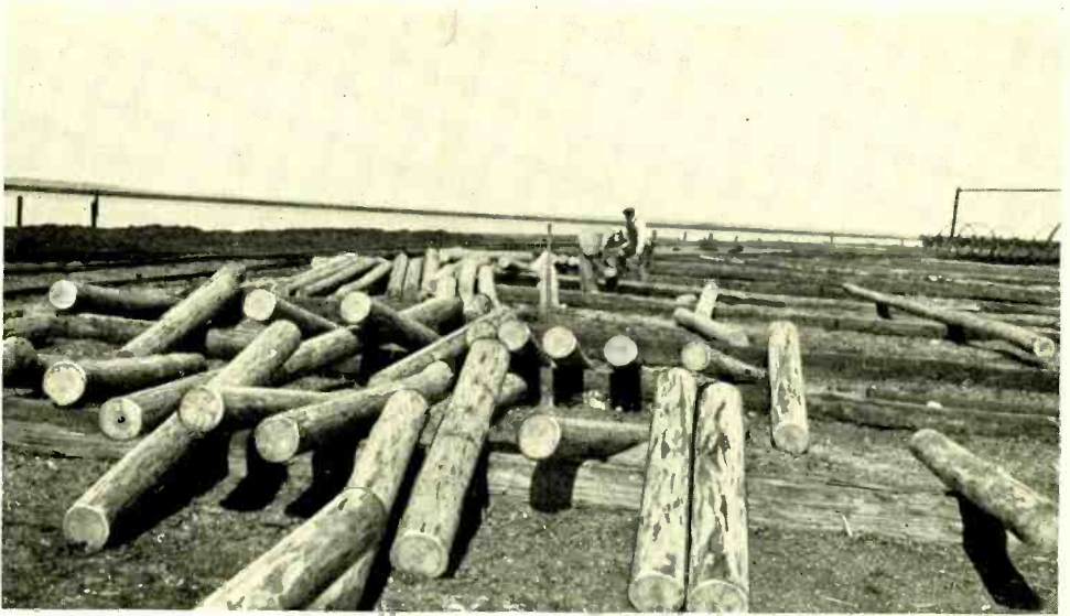
Fig. 2—Poles for use in testing are sawed into eight-foot lengths before they are treated
