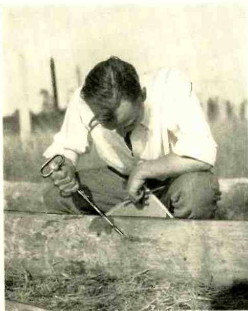
Fig. 6—In this test specimen a rot pocket has formed below the ground line
