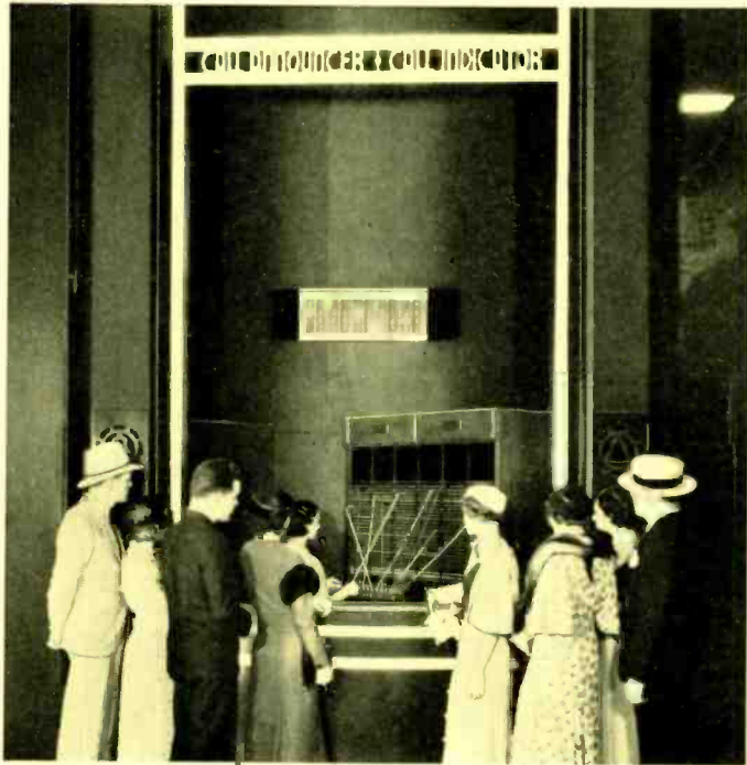
The call indicator and call announcer methods of transmitting dial calls to operators at manual switchboards are shown in one of the niches. Loud speakers mounted behind the Bell System seals let visitors hear the call announcer and the explanations of the operator, who uses a lapel microphone for the purpose. Few visitors will wish to leave the Bell System exhibition without experiencing the acoustic illusions afforded by Oscar, the Dummy with the Microphonic Ears, who is shown below being inspected by John Mills and M. B. Long, prior to the opening of the Bell System exhibit
