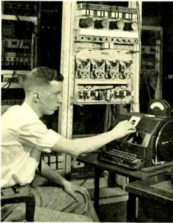
Fig. 2—Four of the repeater units are mounted with their accessory equipment on a single panel for use in the Bell System plant
