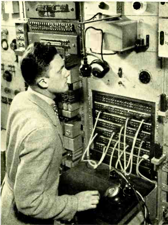
Fig. 1—C. W. Vadersen speaking into the microphone of the speech-synthesizing apparatus
