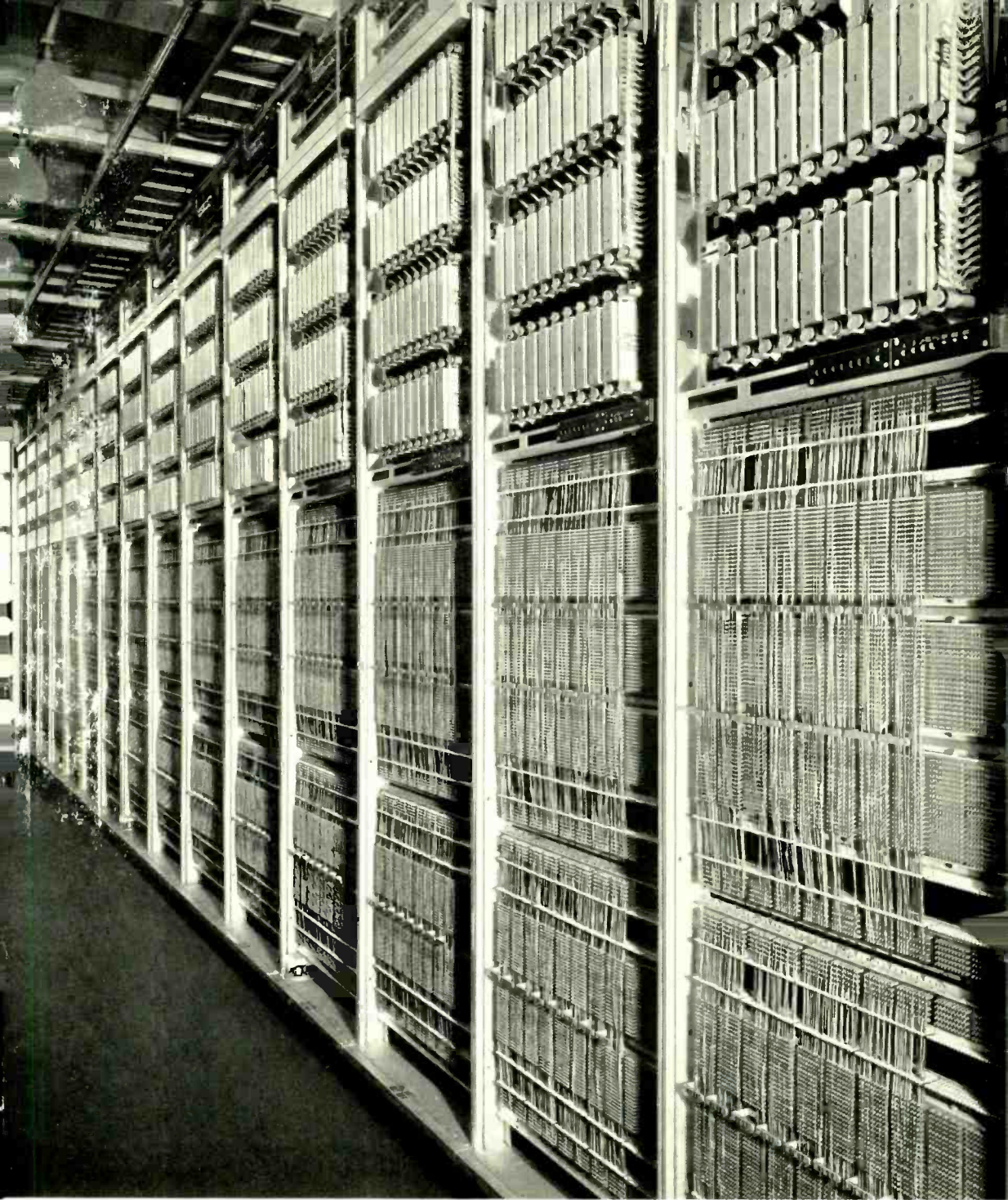
Block relay bays. These are used by the terminating markers for testing lines and determining their location on line-link frames
