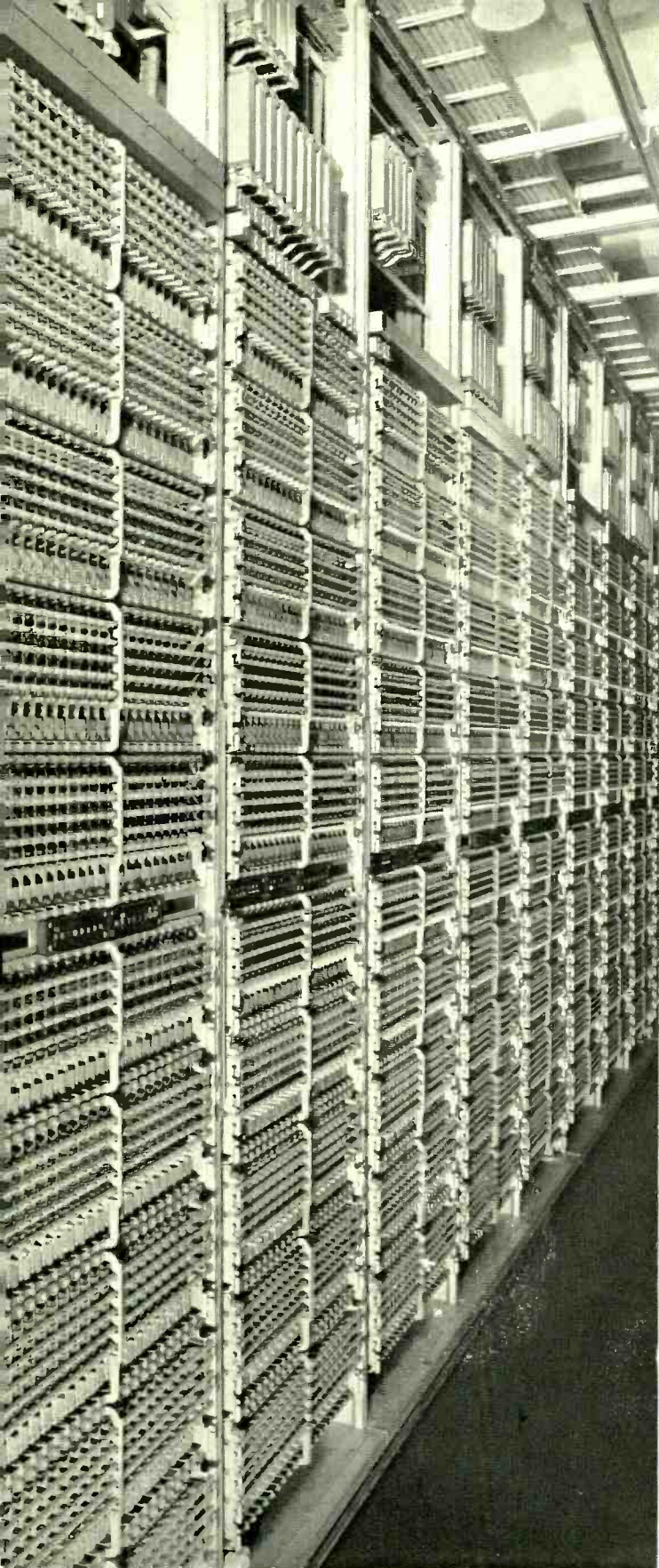
(Opposite page) An originating marker includes three cabinets of U and Y-type relays, at the left and four bays of route relays and cross-connecting terminals
