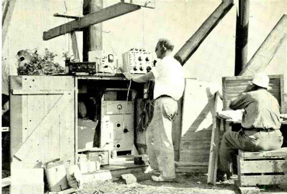
A 1500-foot cable crossing of the Loxahatchee River, on the Charlotte-West Palm Beach system, presented unusual loading problems. The cable is the four-wire disc-insulated type. Loading is being adjusted and the cable is being balanced, in this photograph by W. H. Tidd.
