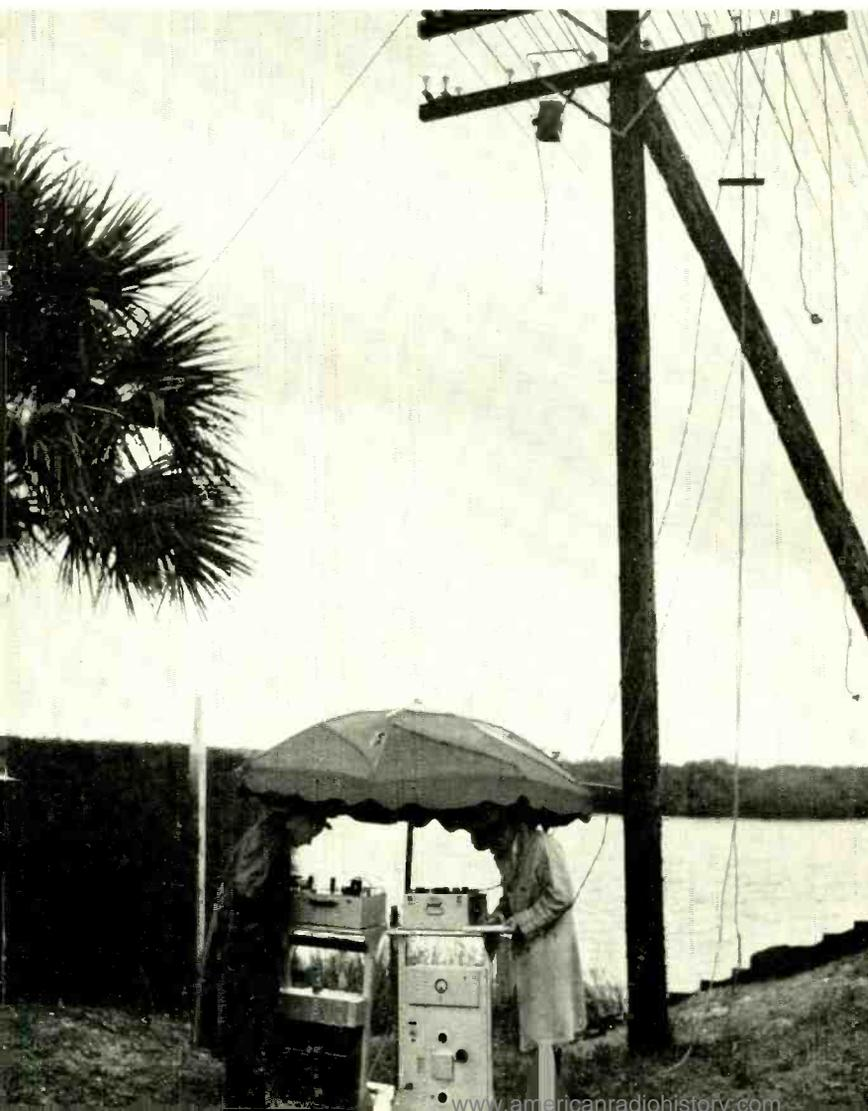
Measuring impedance at a point where transmission irregularities were caused by insulation required to protect the wire from lines cast by wayside fishermen. Photo by W. H. Tidd.
