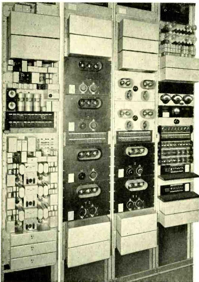
Fig. 1—A C5 terminal, at the left, occupies less than one-third the space required for one of the earlier C-carrier terminals
