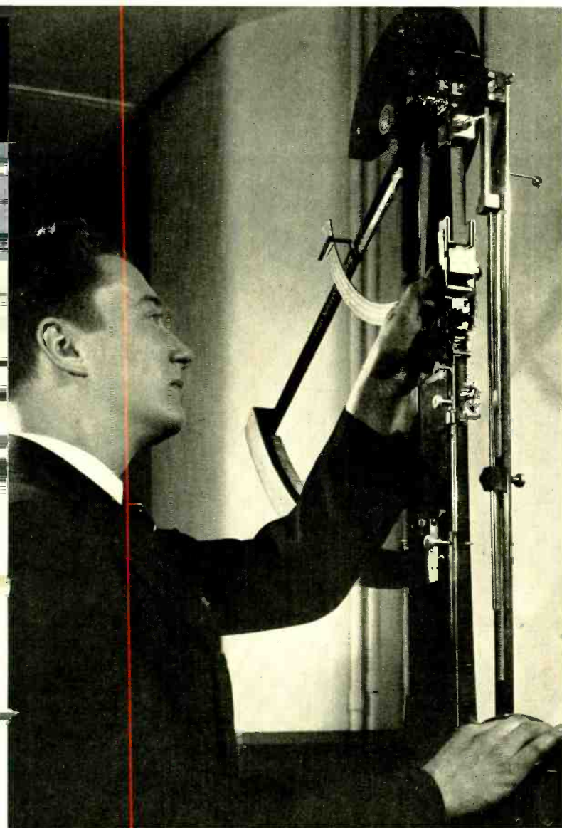
Machine for testing the strength of wet paper, described on page 309
