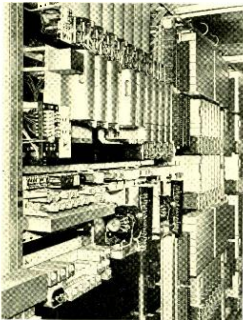
Fig. 2—Miscellaneous equipment mounts on shelves on the same frames as the step-by-step switches
