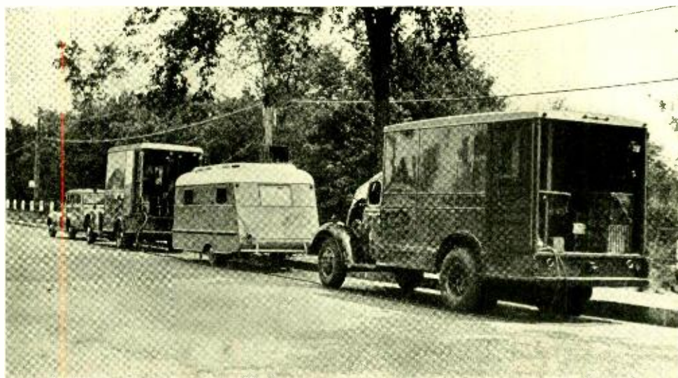
Fig. 1—Mobile equipment for insulation tests on aerial cable
