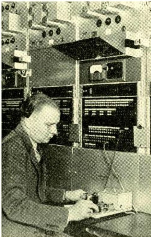
Fig. 5—Monitoring is commonly done at the amplifier bays, and in this position, at the Omaha toll office, the cue lamps and keys are in the jack multiple
