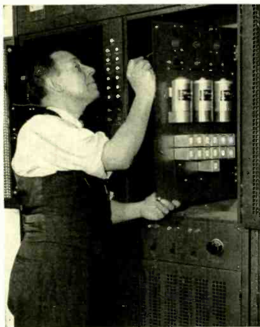
At Rutherford, New Jersey, WHN has recently placed in operation its new 50,000-watt radio transmitter, developed for Western Electric by the Laboratories. Top—Bank of 18,000-volt rectifier tubes. Lower left—J. C. Herber adjusts a relay in the control unit. Lower right—Plate tuning and harmonic filter inductances, and condensers in the 50-kw amplifier unit
