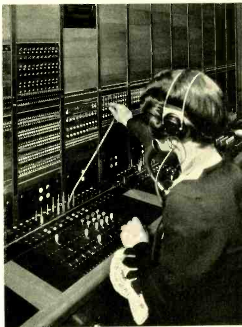
Fig. 2—A typical sender-monitor position of the 13C board
