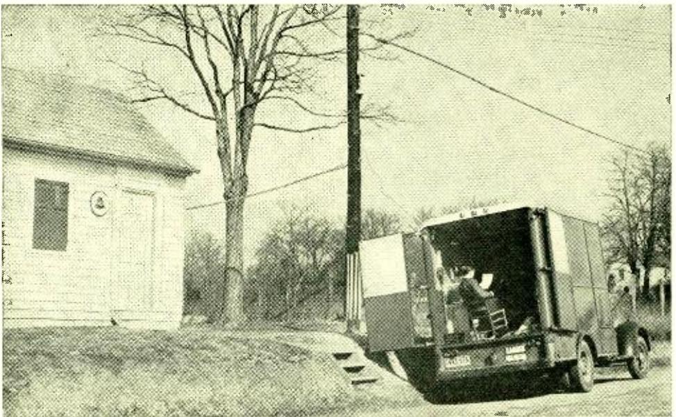
*Bell Laboratories test truck making transmission measurements on power-line carrier circuit just outside a rural central office*
