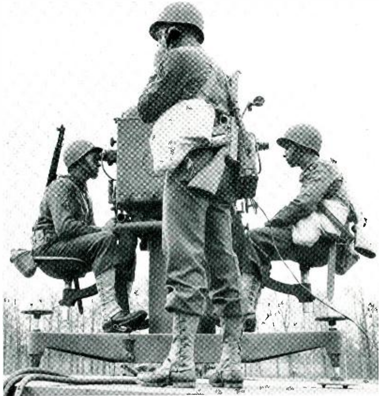
The tracker of the Director as set up for demonstration at Murray Hill. One soldier orients the telescopes in elevation while the other orients them in azimuth by turning the entire tracker ahead
