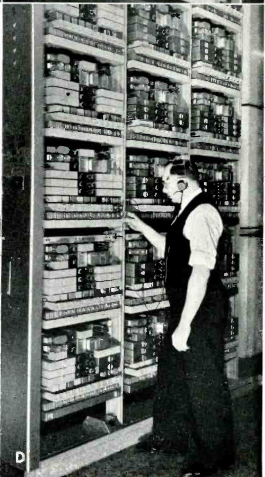
Fig. 2A—Dial senders and marker connectors in the Philadelphia crossbar toll office
