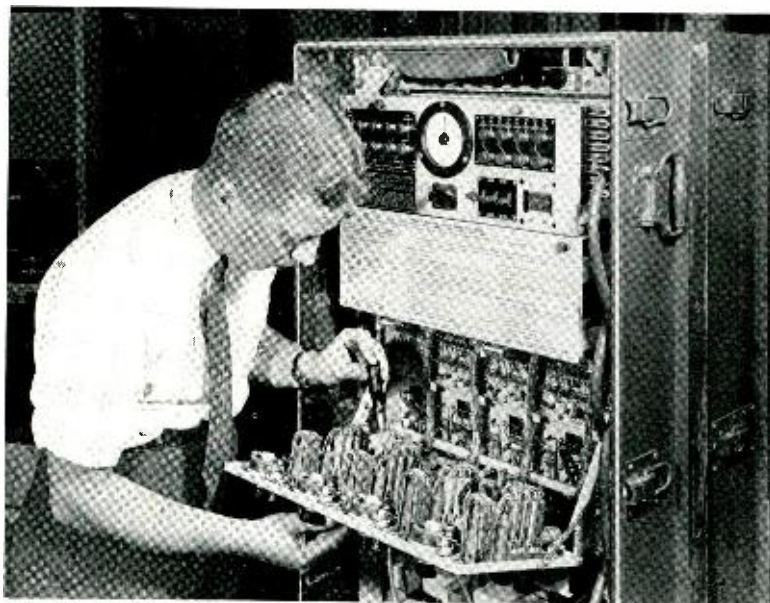
Fig. 5—Panels carrying various components of the circuit may be tipped forward to give access to all apparatus and wiring
