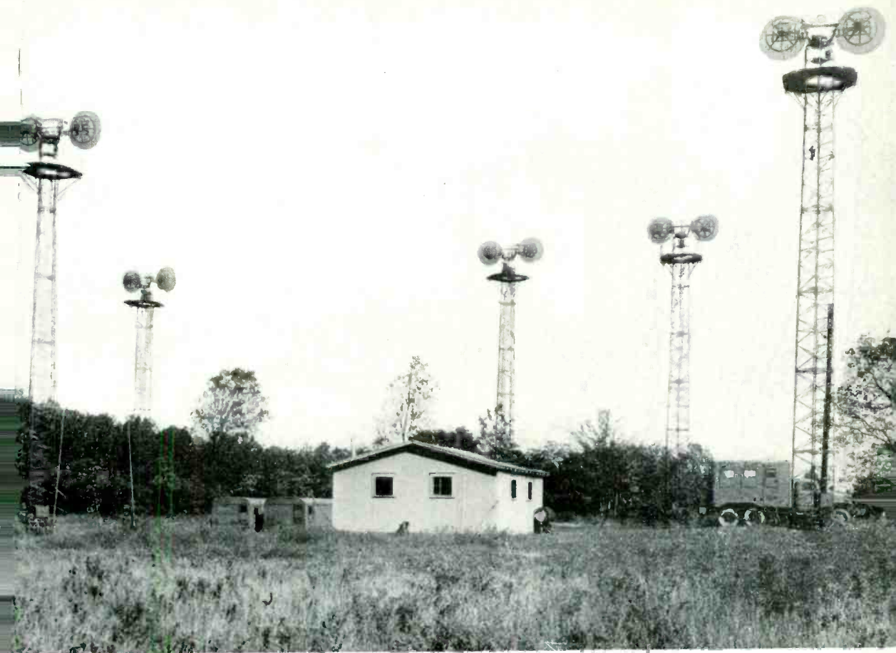
AN/TRC-6 antenna structures at Neshanic, New Jersey
