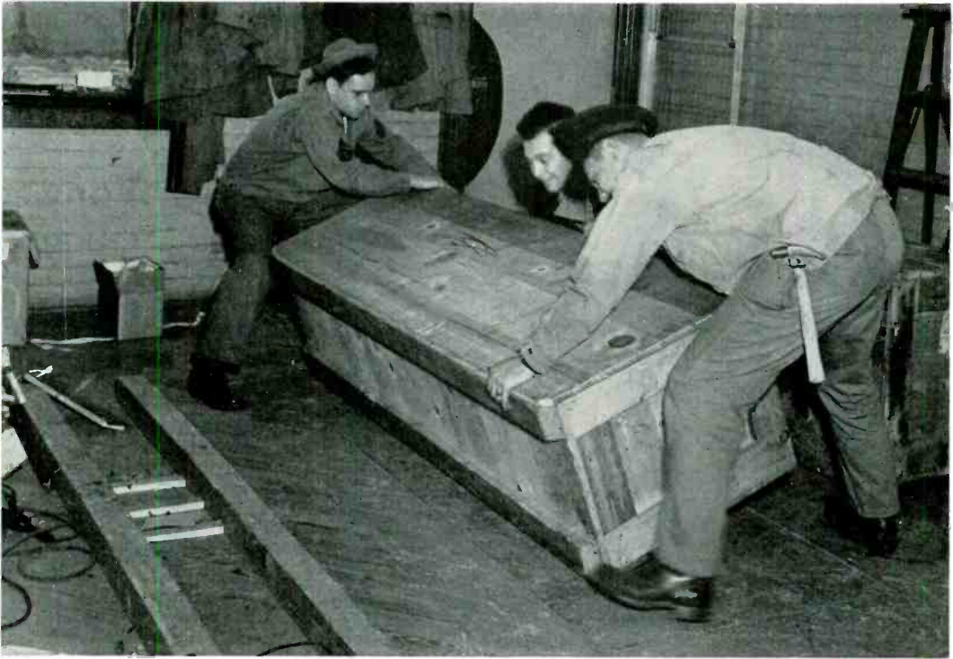
Unpacking a cabinet from the shipping case. The cabinet will be set on the parallel timbers at the left and the wiring run in the trough between them
