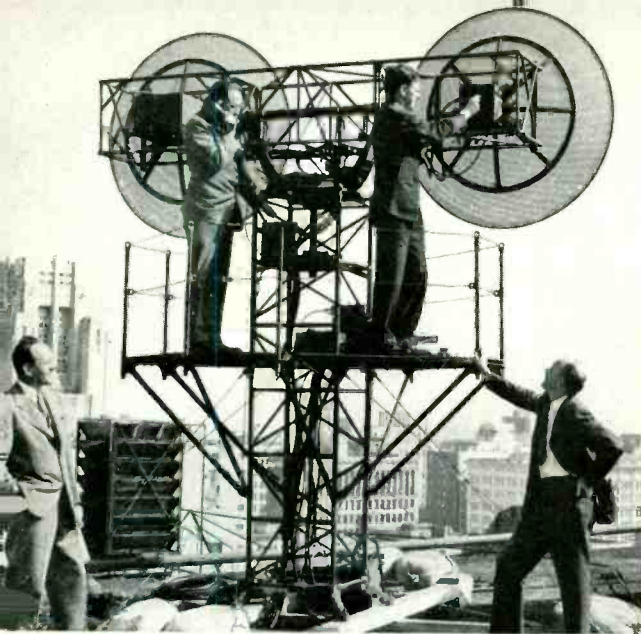
Microwave antenna array at the Los Angeles terminal of the Southern California Telephone Company's eight-channel radio system to Catalina. On the antenna platform are L. R. Montfort and Nean Lund
