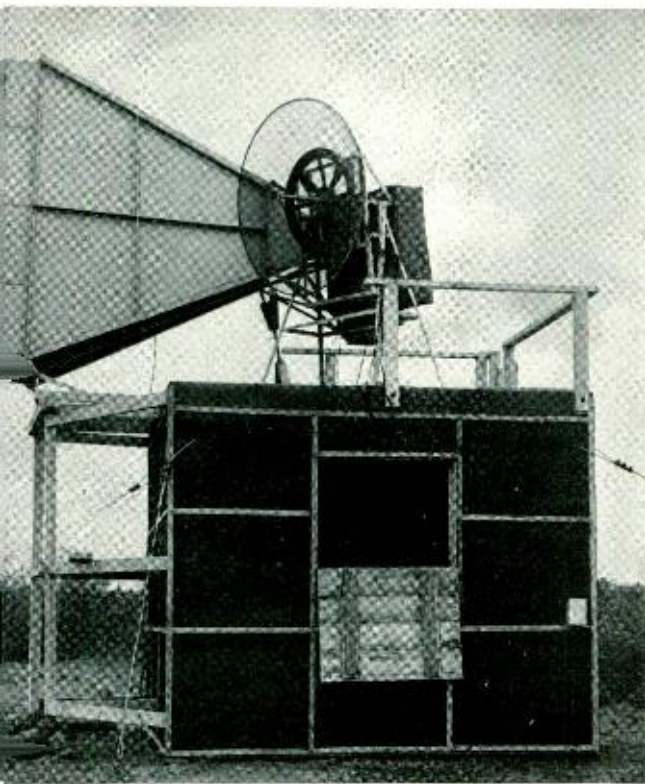
Microwave relay station on Crows Nest Mountain at West Point used in the first two-link radio television system operated commercially by the Bell System. Three of Army's home games were televised by the NBC and broadcast from New York City
