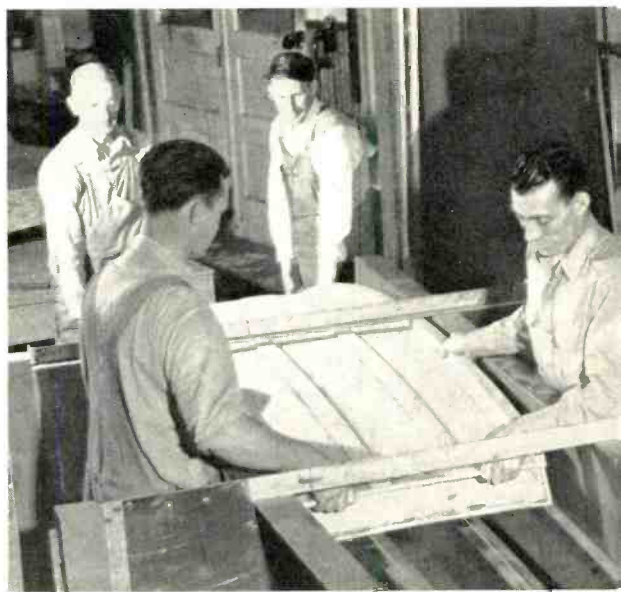
One of the steps in the construction of an experimental plywood horn-reflector antenna for microwaves. Left to right, W. E. Thomsen, C. A. Davison, O. E. Larsen, and J. Morrell removing a section of the reflector surface from a metal jig.
