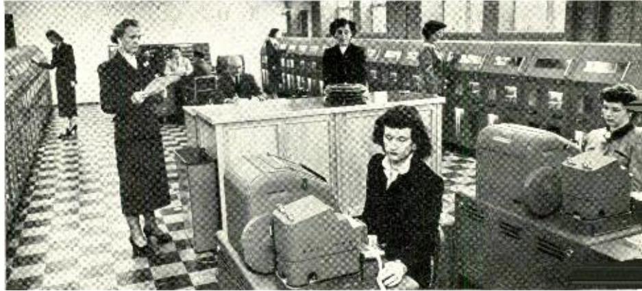
Switching center of the Ford 81C1 system. Rows of reperforator-transmitters mounted two to a machine cabinet are at left and right. In the extreme rear is the control board.
