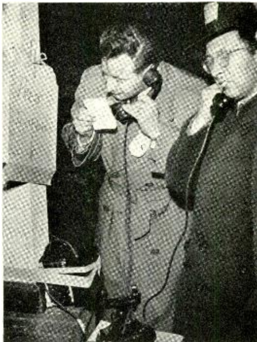
Reporters telephoning stories of Long Island wreck from two emergency handsets.
