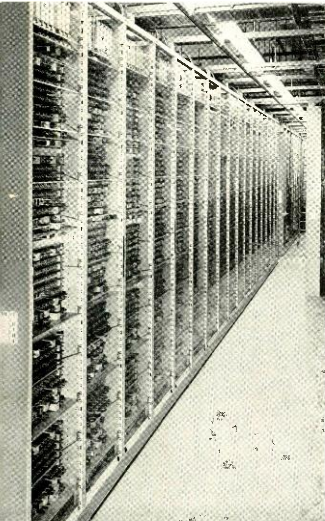
Fig. 4—A line of originating register bays in the Towson office. The distribution of calls to these registers is under control of the circuits in the marker that is described in this article.
