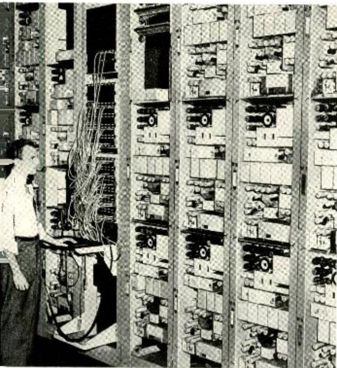
Fig. 7—An installation of repeaters for local wire television networks in a central office.
