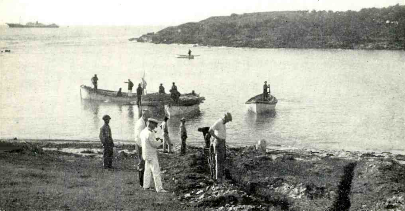
HISTORIC FIRST, 1924 — Dr. Buckley, center foreground, looking at one end of the 120 nautical-mile trial-length of loaded telegraph cable at Bermuda.
