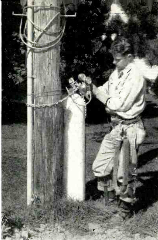
Fig. 4—Charging the cable from a tank of Freon.
