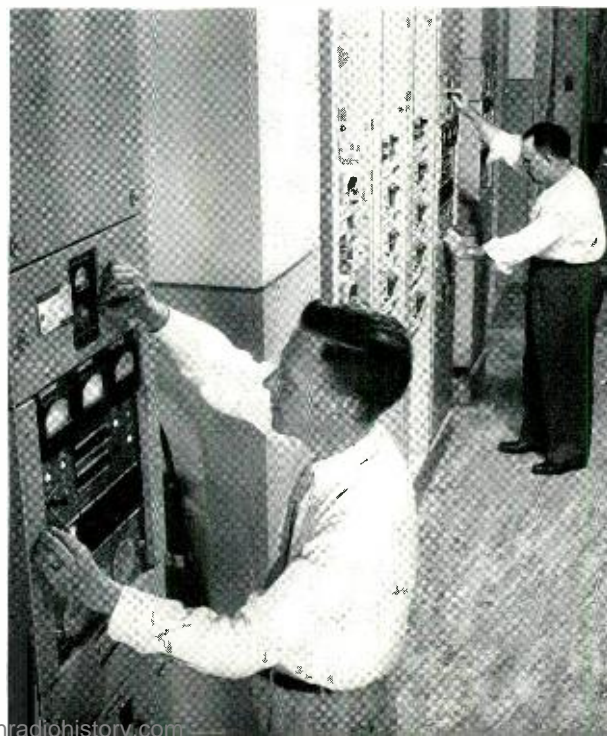
Fig. 3 — The author (left) and O. D. Grismore observing line current at the power control bays in an L3 terminal.
