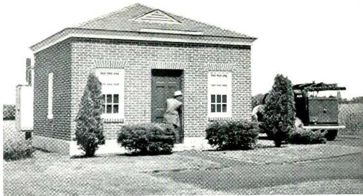
An L3 auxiliary repeater hut at Scotch Plains, New Jersey.
