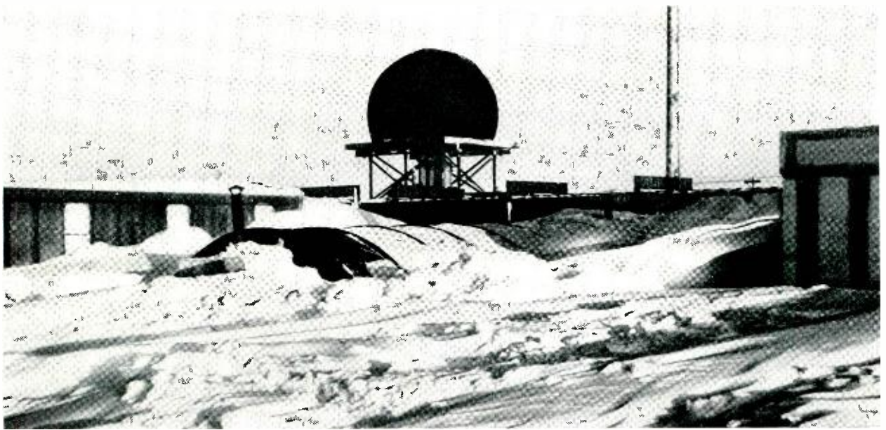
Inside the mushroom-shaped rubber dome is a radar antenna that is one of the experimental units in the Distant Early Warning Line in the Barter Island area in Alaska.
