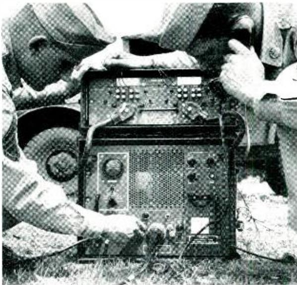
*Four-channel cable terminal. AN/TCC-3.*
