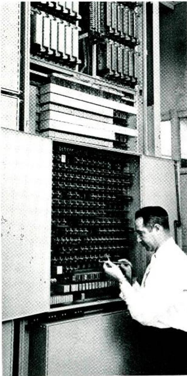
Fig. 2 — S. J. Argerie is shown checking the relays of a sender link controller. The controller connector is in the top half of the bay, with some of the associated senders in the bay to the left.
