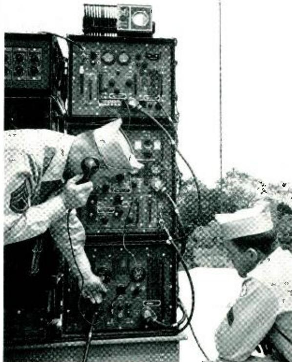
Vital military messages can now be telephoned over the system via terminals and both attended and unattended cable repeaters, and, where conditions merit, transferred at will to radio portions of the overall network. Various lengths of cable and various numbers of radio stations can be quickly interchanged or interspersed. By proper grouping of equipment, communications distances of 800 to 1,000 miles and greater can be achieved.
