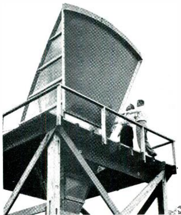
Fig. 4 — L. C. Tillotson (left) and A. T. Corbin inspecting glass fiber cover on face of horn reflector antenna at the Holmdel Laboratory.
