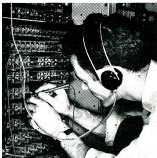
Fig. 6 — The author inspecting code register relays in Laboratories installation of No. 5 crossbar outgoing sender.
