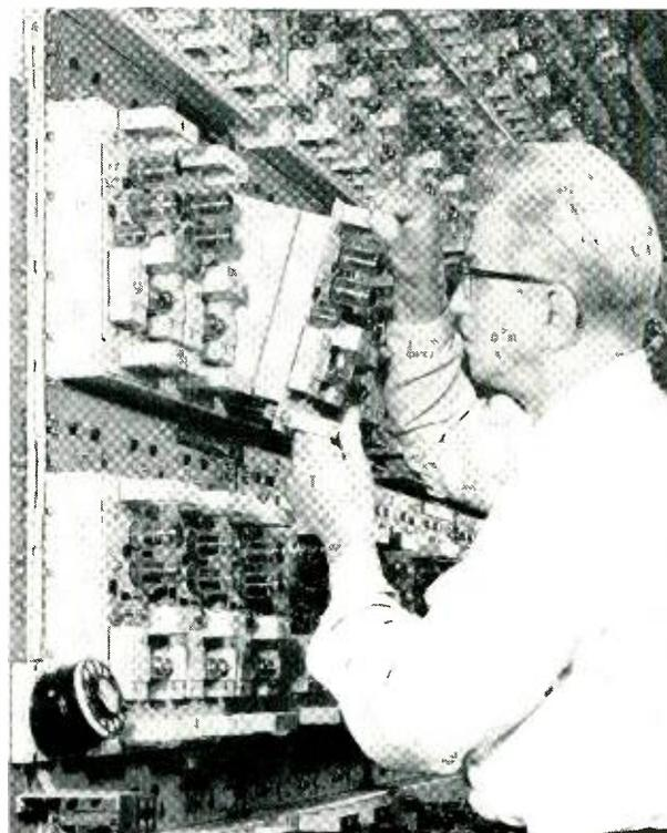
Fig. 3 — Peter A. DeCarlo removes a channel terminal from the bay.
