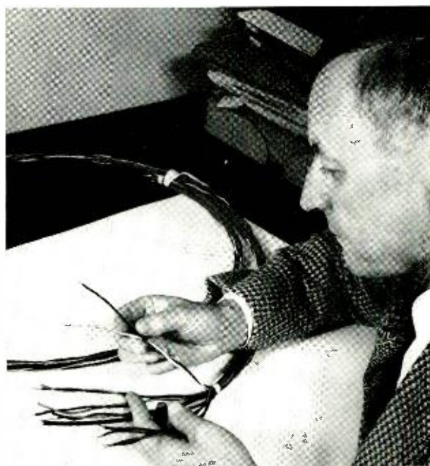
Fig. 1—A. P. Jahn of Outside Plant Development demonstrates how any one of the six pairs of conductors is easily identified by color.
