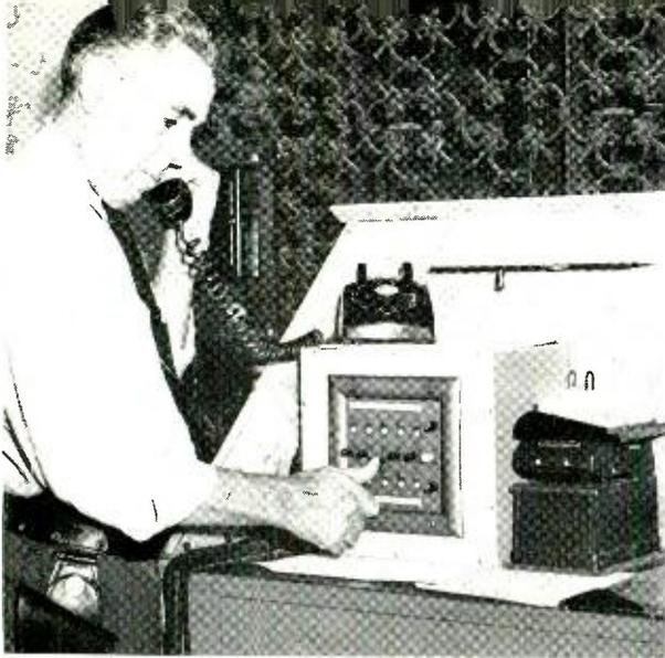
Fig. 2 — 101 key equipment used for night service at the Laboratories in New York City.
