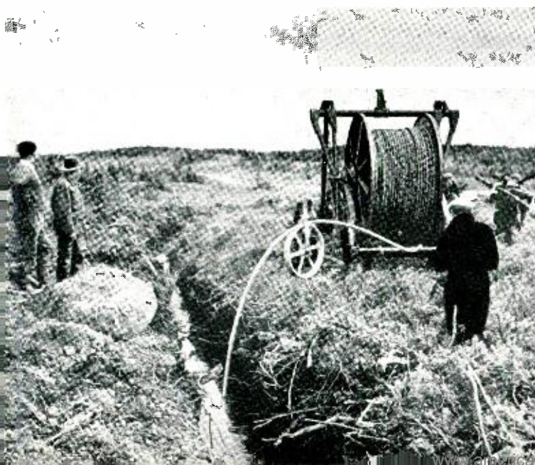
Fig. 4—Land cable being laid between Clarenville and Terrenceville in Newfoundland.
