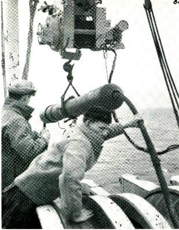
Fig. 3 — A British rigid repeater is laid with the cable in the waters of Cabot Strait.
