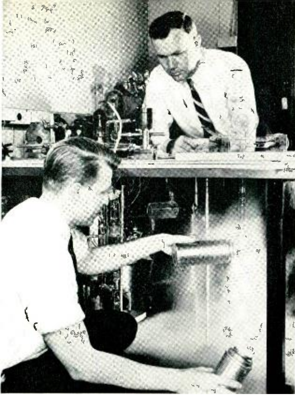
H. Kraft (left) and K. B. McAfee, Jr., engage in measurement of gaseous diffusion through glass and high-alumina ceramics. Mr. Kraft is pouring liquid air into cold trap of high-vacuum apparatus.
