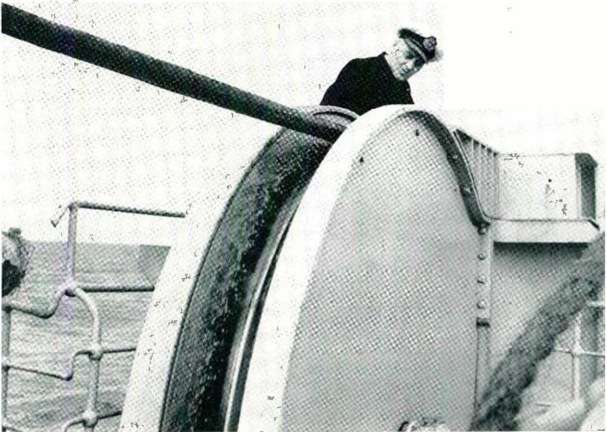
*The transatlantic cable shown here paying out off the stern of the cable-laying ship H.M.S. Monarch. The fifty-one repeaters had to be*
