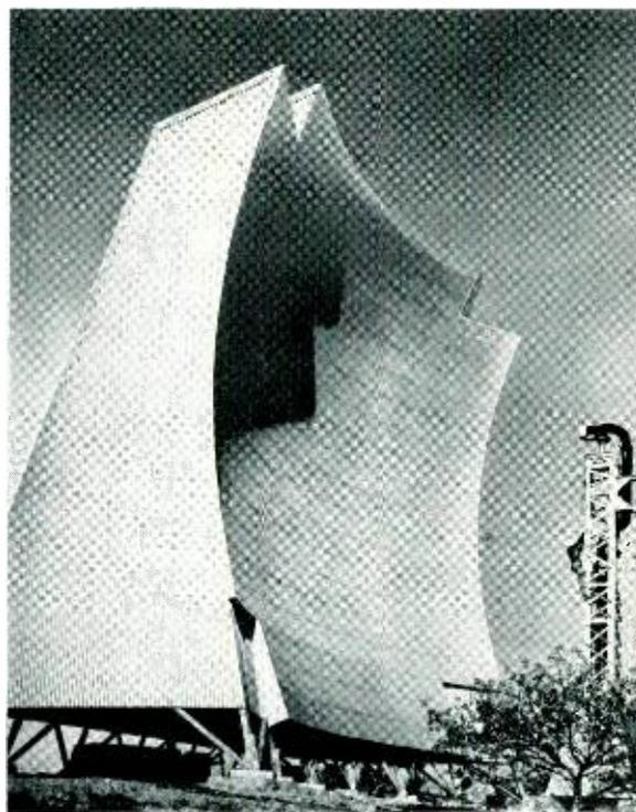
*DEW Line terrain sometimes presents difficult or unusual transmission problems. Here, the lateral system uses higher-powered, sixty-foot antennas.*
