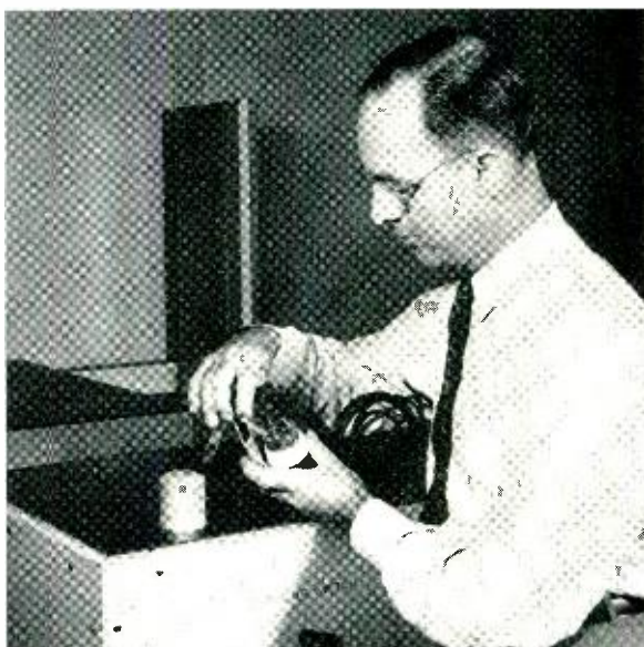
J. B. Hays checks spacing of carbon blocks on the 118A protector. Gap of 0.02 inch arcs at 2000 volts.
