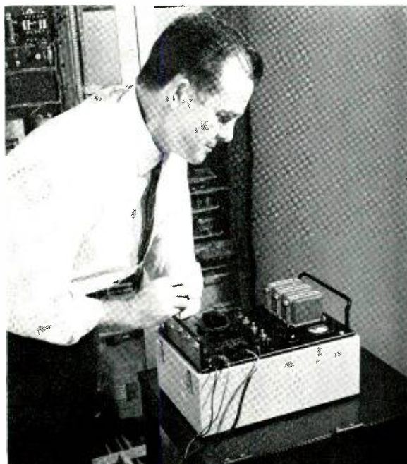
E. K. Ward of Pacific Telephone and Telegraph Co. adjusts a gate threshold on a statistical ammeter.
