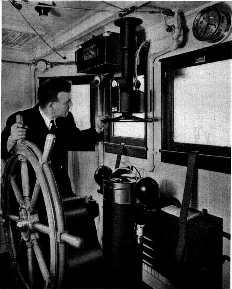
Fig. 2—Marine radio compass installed on a trawler.
