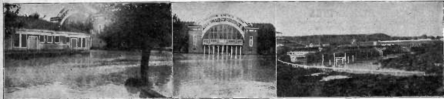
WHAT FLOOD DID TO PLANT OF MIDLAND EMPIRE FAIR, Billings, Mont., when a cloud-burst came down Alkali Creek on June 11. Left to right: Secretary's office with auditorium in background, dark line around building marking high water stage. Front view of Auditorium day after cloud-burst. View of race track in front of grand stand, rough masses on both sides of white fence being hail seven feet deep, darkened by debris washed down with it.
