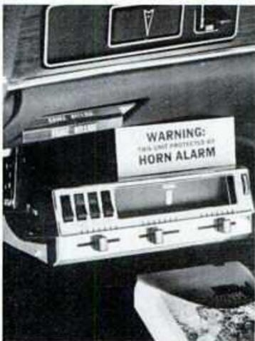
ANTI-THEFT ALARM is incorporated into Channel Master's Model 6292 8-track car player. Any attempt to remove unit sets off auto horn. List is under \$70.
