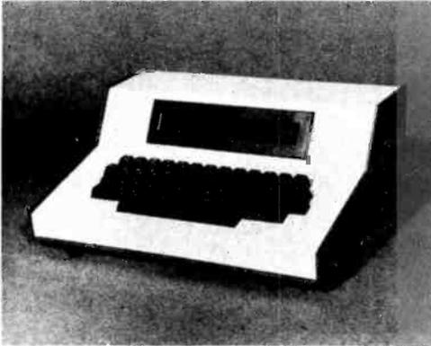
The Transactor III data terminal utilizes a microprocessor in its design. Features available include synchronous or asynchronous communications line support for both dedicated or polled
